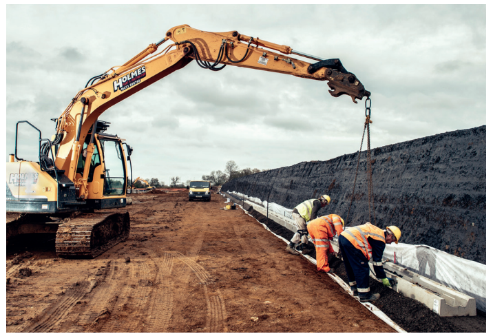
Section trough single wall earth bund
